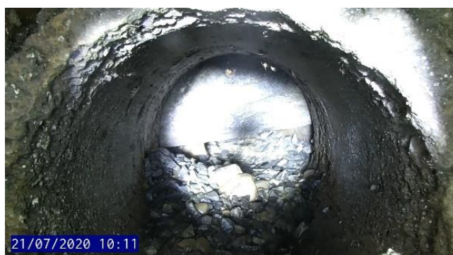
Examples of blocked pipes
